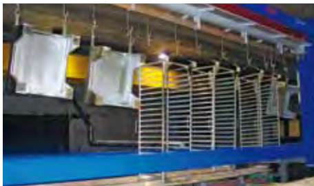
- TELAI IN ZINCATURA - ELECTROLYTIC GALVANIZING OF METAL STRUCTUREE
