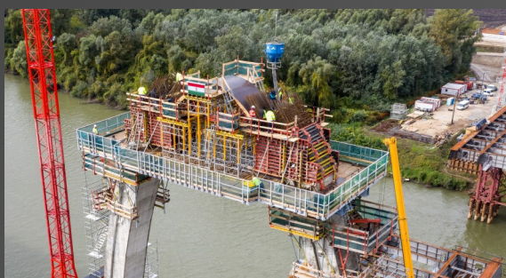
Bridge over Tisza M44 - production and mounting of auxiliary structures and handrails
