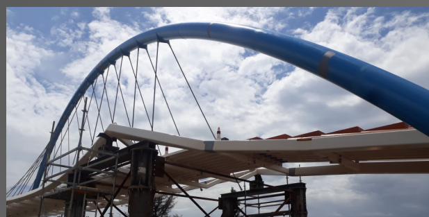
Bridge in Györszentiván - Production of access ramps
