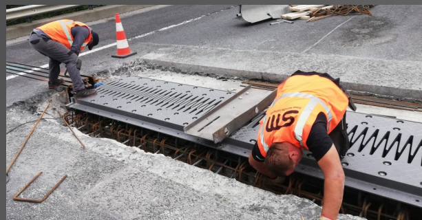
Highway M1 - Production and installation of XTEND joints
