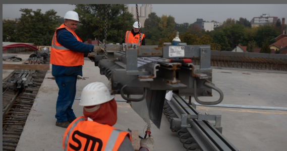
Bridge „Y” in Miskolc - installation of bearings and joints type MAURER
