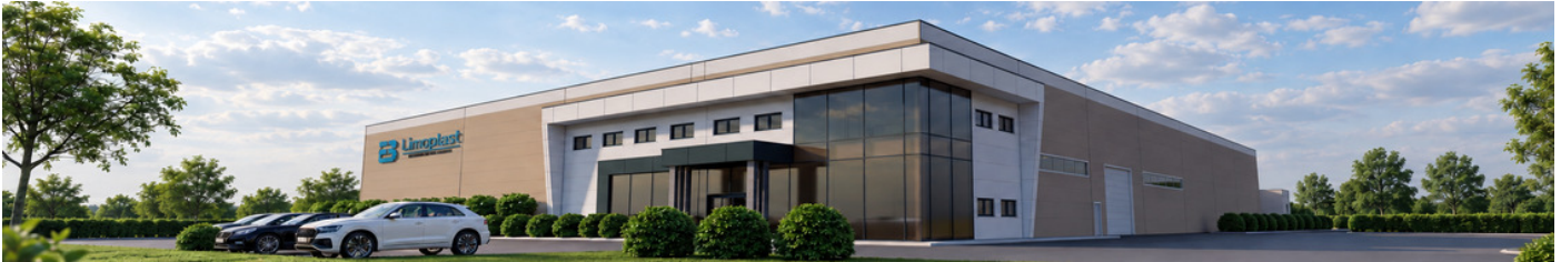
Architectural visualisation - new production facility in the Industrial Zone Lugovi, Šamac
