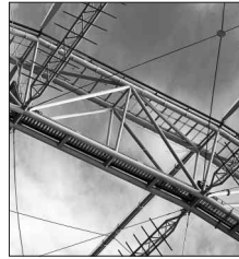
Cargo-Lifter Brand, Windverband
