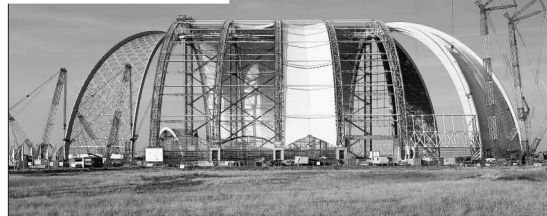
Cargo-Lifter Brand, Windverband
