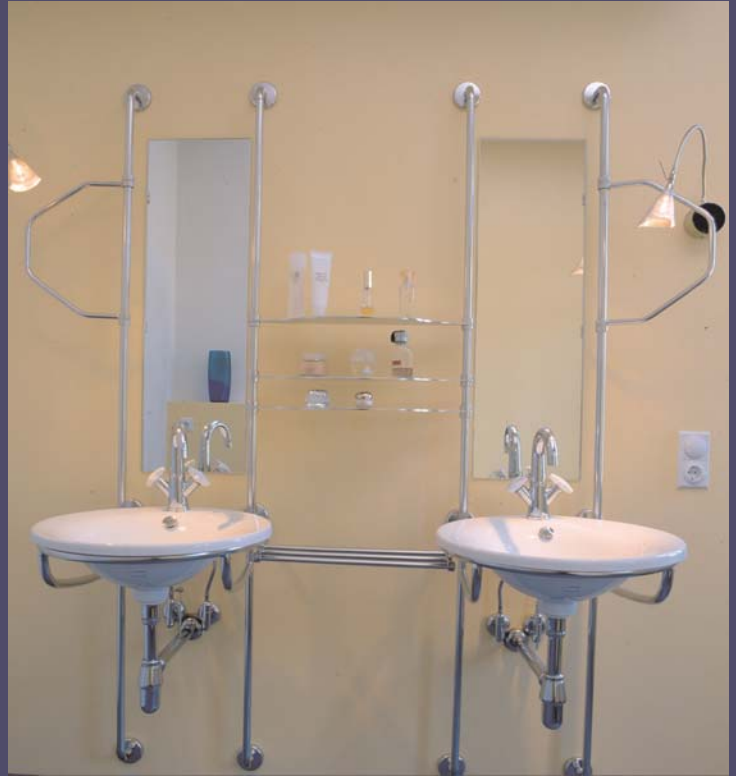
Individual staircases and handrails are looking light and transparent. And an especially furniture in the bathroom is also a good investment.
